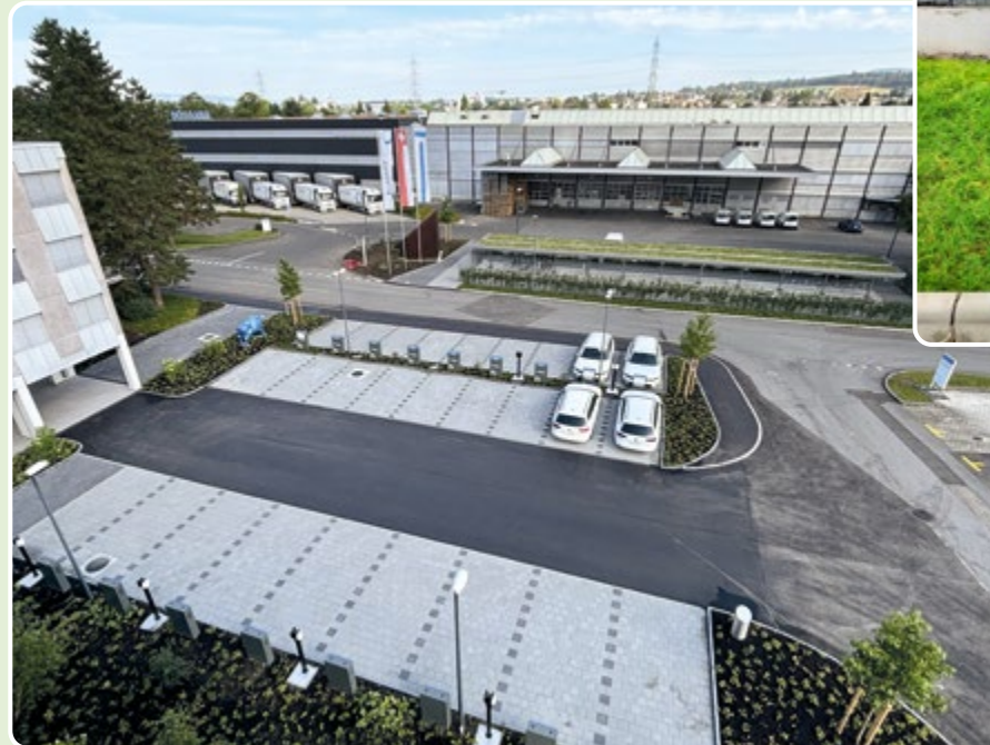
Charging infrastructure: Bossard Switzerland – The visitor parking lots now offer charging infrastructure that is powered by 100 percent renewable electricity.
