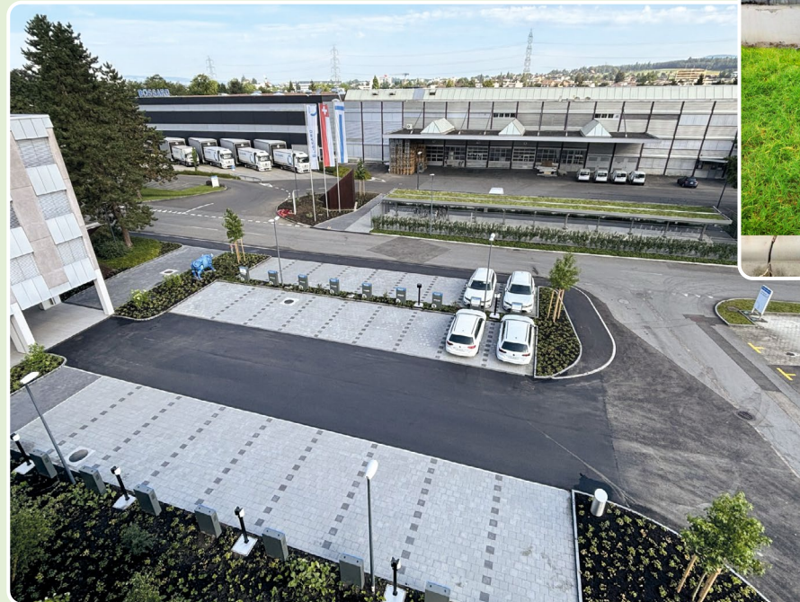
Charging infrastructure: Bossard Switzerland – The visitor parking lots now offer charging infrastructure that is powered by 100 percent renewable electricity.
