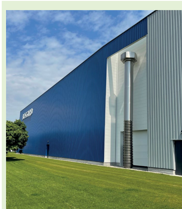
Energy-efficient: Bossard's warehouse in France.
